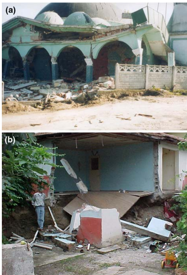
Fig. 15 Normal fault east of Gölcük, Kocaeli, Turkey 1999 earthquake—Denizevler: a Mosque resting on flexible foundation (isolated footings), and b 1-story cinder-block building (photo from Youd et al. 2000), directly founded on the ground (very flexible foundation). Both buildings were subjected to about 1.5 m differential displacement and partially collapsed
