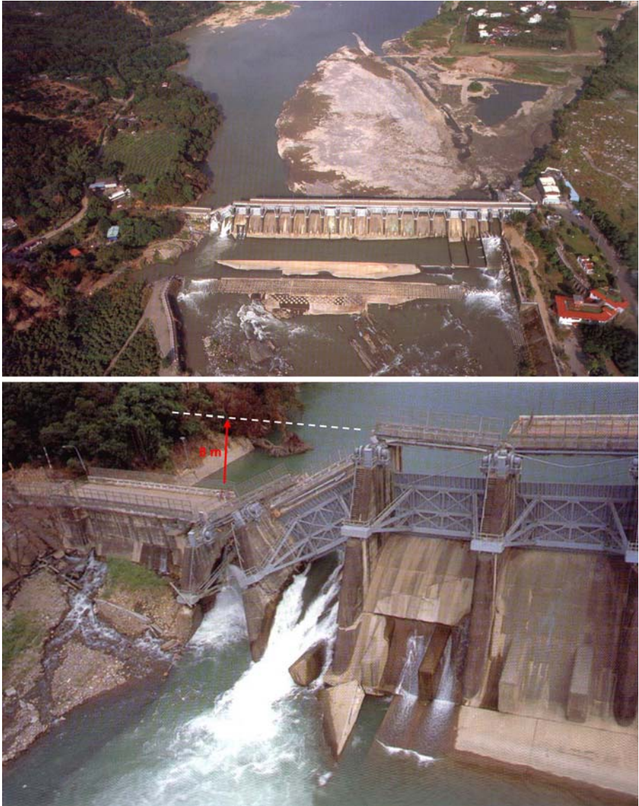
Fig. 18 Chelungpu thrust fault, Chi-Chi, Taiwan 1999 earthquake—Shih-Kang Dam. The fault rupture passed through the northern part of the dam with an upthrust of about 8 m, destroying spillways and gates. Due to its length of 700 m, the dam behaved as a flexible structure, practically following the imposed deformation (photos adapted from Hwang 2000 )
