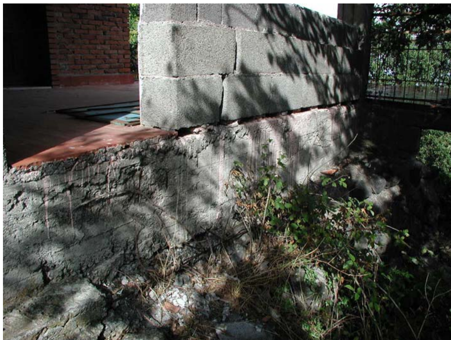
Fig. 5 Mt. Etna—1-story building of Fig. 4. Detail of the reinforced concrete ring beam around the raft foundation
