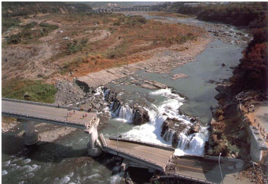
Fig. 19 Chelungpu thrust fault, Chi-Chi, Taiwan 1999 earthquake—Fung-Yan City. The fault rupture passed through the south abutment of the Bei-Fung bridge with an upthrust of about 7 m, causing the collapse of two spans and the development of a small, but impressive, waterfall (photos adapted from Hwang 2000 )
